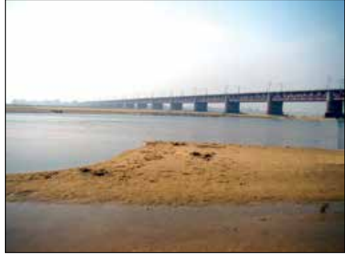
Fig. 1. Downstream river Sone at Koilwar near Arah
